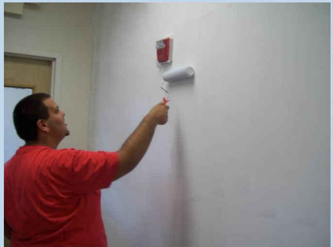
Josh helps to refurbish QFI.
